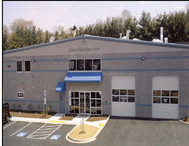
WARNER CONST. GIVENS COLLISION REPAIR CENTER
