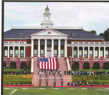
RCD INC. ELECTRICAL JOHN HANDLEY HIGH SCHOOL HISTORIC
